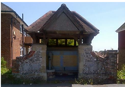
Willington Village Pump House (An existing locally listed building)
